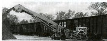
UNLOADING AGGREGATE FROM RAILCAR
